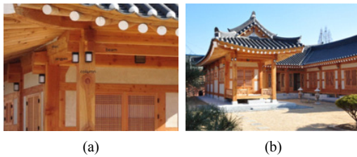
Fig. 1. (a) Photograph of Eum-pyeong hanok in Korea, (b) Close-up view of part of a hanok and its elements.
