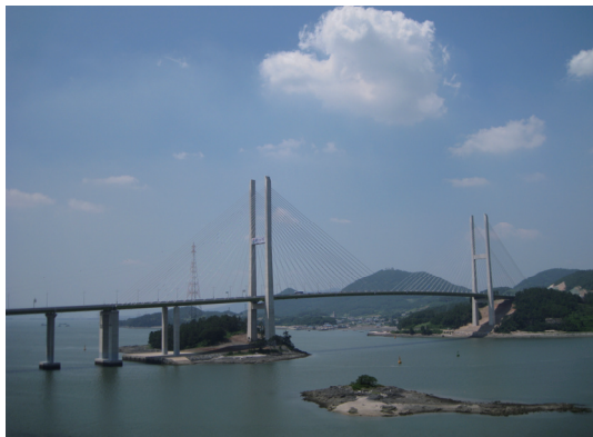
Fig. 1. A panorama of cable-stayed bridge (subject of study)
