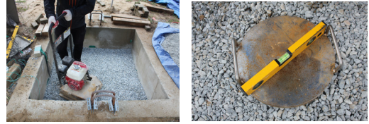
Fig. 7. Ground compaction
