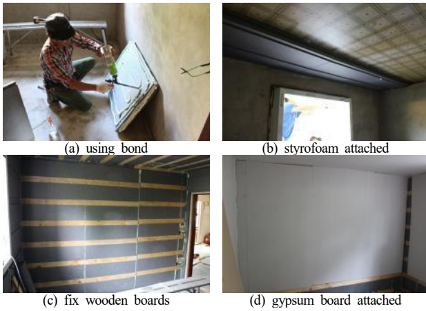
Fig. 2. Insulation work using styrofoam
