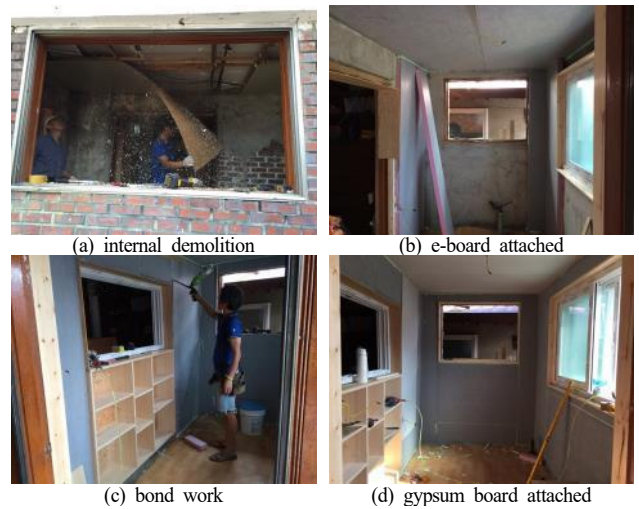
Fig. 5. Insulation work using e-board
