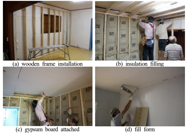
Fig. 8. Insulation work using Glass wool
