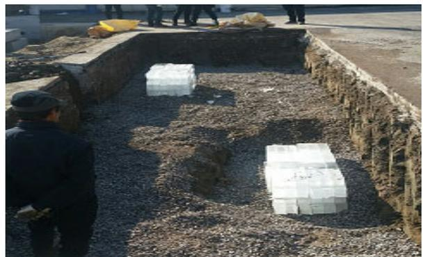
Fig. 11 Artificial Cavity Installation
