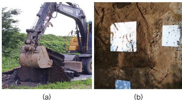
Fig. 7 Pavement Removal & Installing Styrofoam
