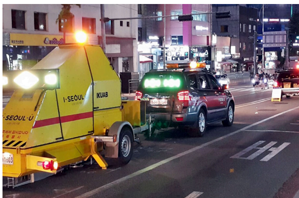
Fig. 3 FWD Test at a Section with Cavity
