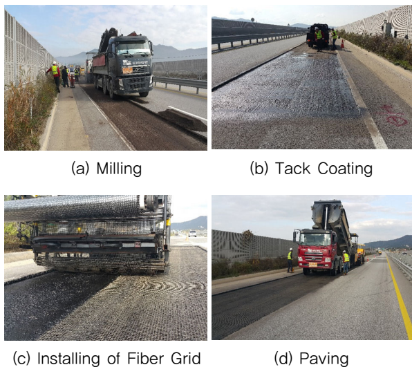
Fig. 4 Construction of Fiber Grid Reinforced Asphalt Pavement
