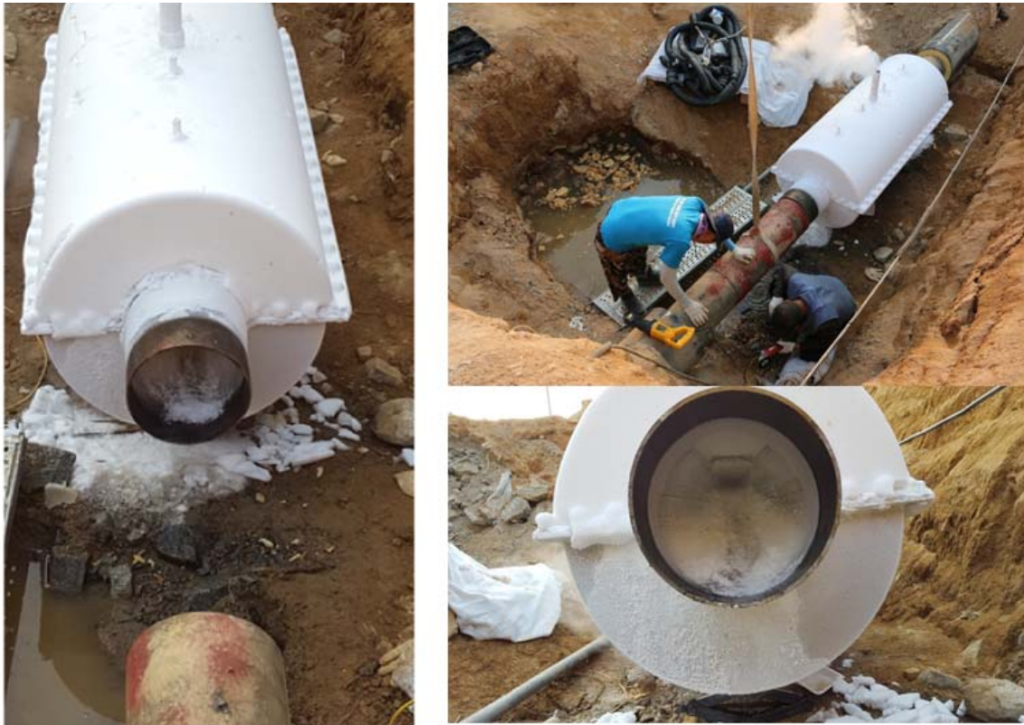
Fig. 7. Ice-Plug for freezing seal isolation in pre insulated heat transport pipe(300A) at KDHC
