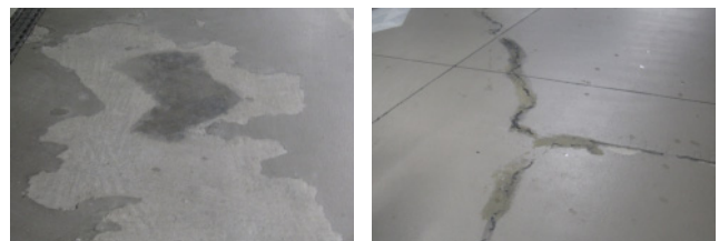
(a) Delamination
