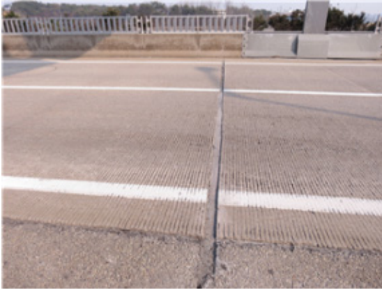
Photo 3 Expansion joint construction(On-site)
