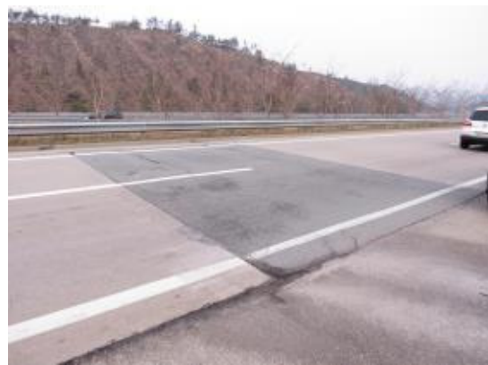
Photo 4 Replacement with asphalt(On-site)
