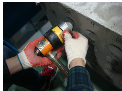
Photo 5 Simplified pullout test including load cell
