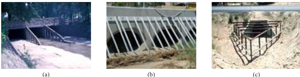
Fig. 1. Debris Reduction System(FHWA, 2005) (a) debris fins (b) debris racks (c) debris deflectors
