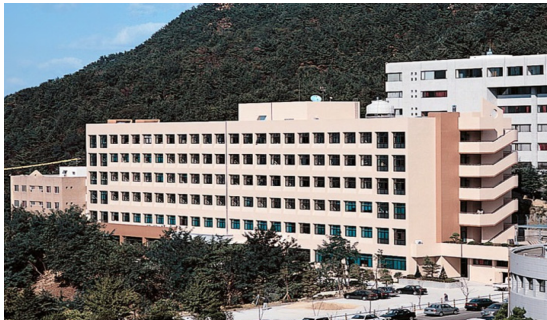
Fig. 4 Test-bed a) Common building
