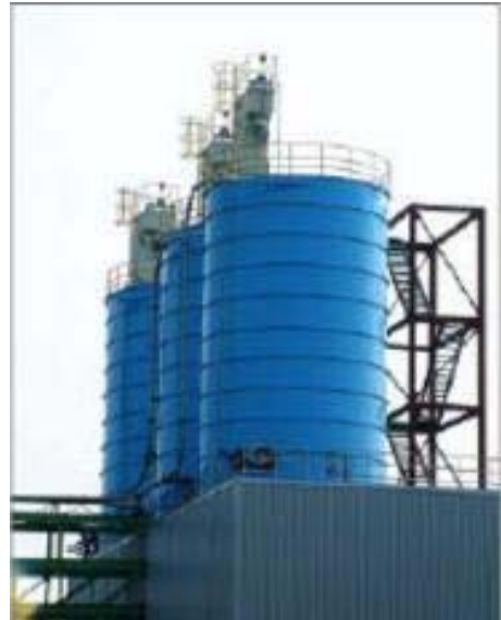
Fig. 3. The form of installing cylinder type structure.
