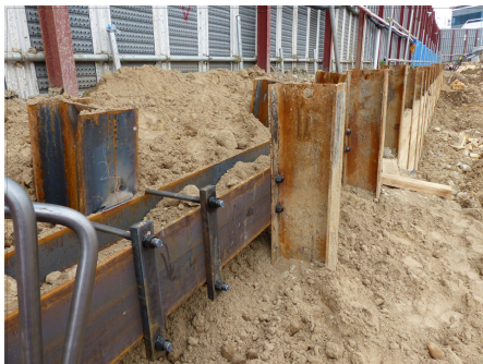
(a) Head fixing structure
