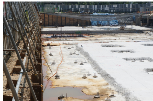
(b) Construction site after excavation
