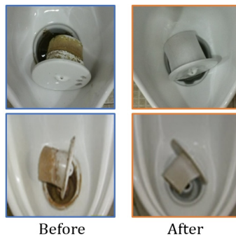
Fig. 7 Photograph of scale removal of toilet urinal.
