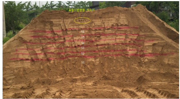
(b) Construction of slope models
