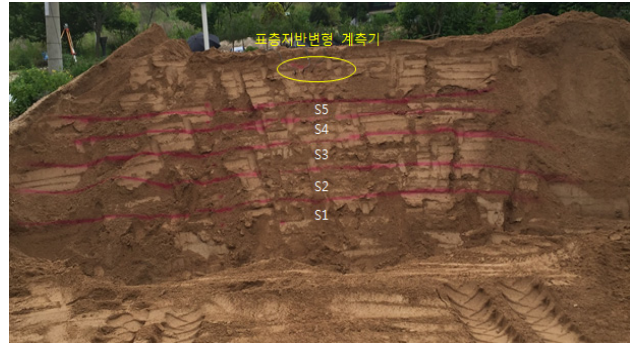
(b) Construction of slope models
