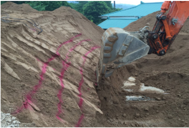
(a) Excavate soil
