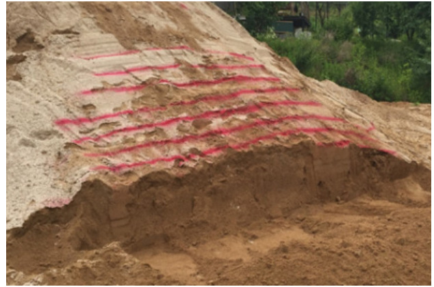
(b) Construction of slope models
