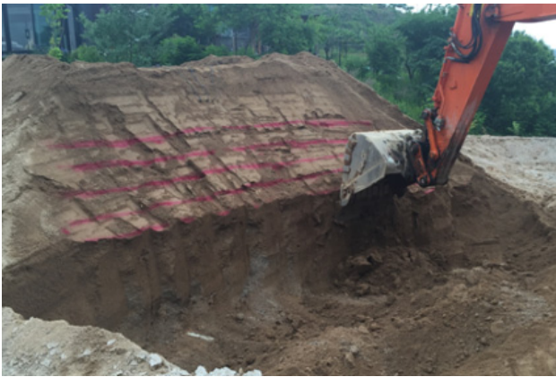
(a) Excavate soil
