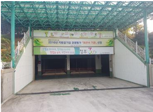
FIGURE 3. The upper part of Jisan sewage disposal plant
