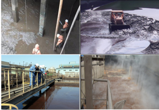
Fig. 1 General cleaning work methods and cistern environments
