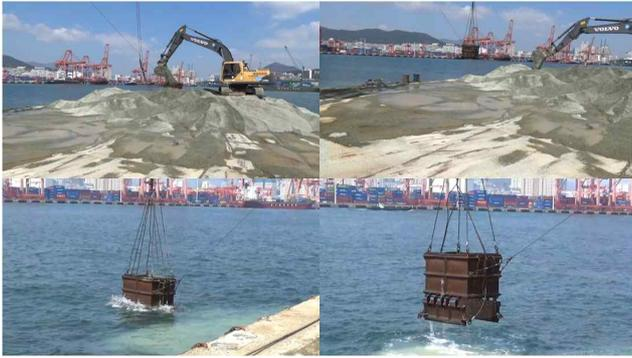
Fig. 4 Digital image of equipment and cap construction using setting barge with clam shell
