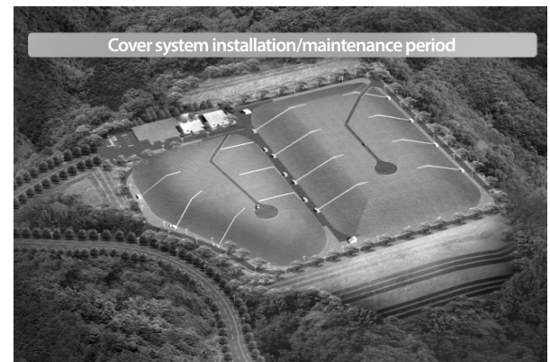
(c) The 2 nd stage near surface disposal facility after closure : monitoring for cover system and disposal vault performance
