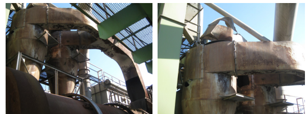
Figure 7. Damaged cyclone.
