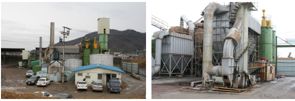
Figure 3. Asphalt plant that explosion broke out.
