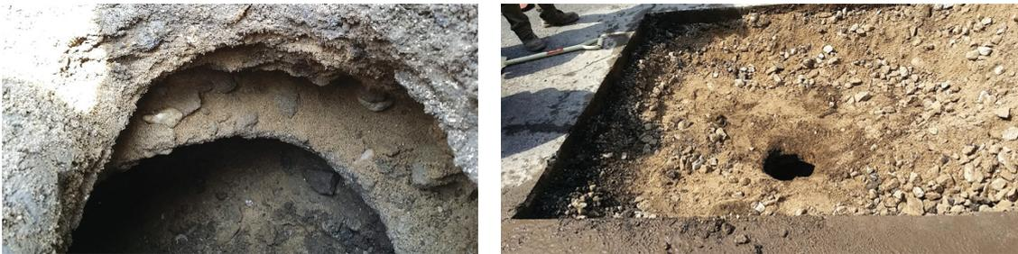
Fig. 1. Example of Ground cavity (Choi et al., 2015)
