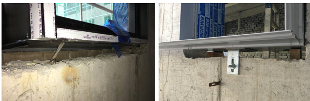
Fig. 3 Junction by anchor-bolt and fixed hardware
