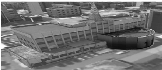
Fig. 1. The picture of actual Building
