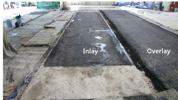
Fig. 6 Asphalt Overlay Placement
