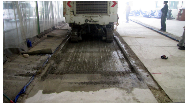
Fig. 5 Concrete Milling (7cm Deep)
