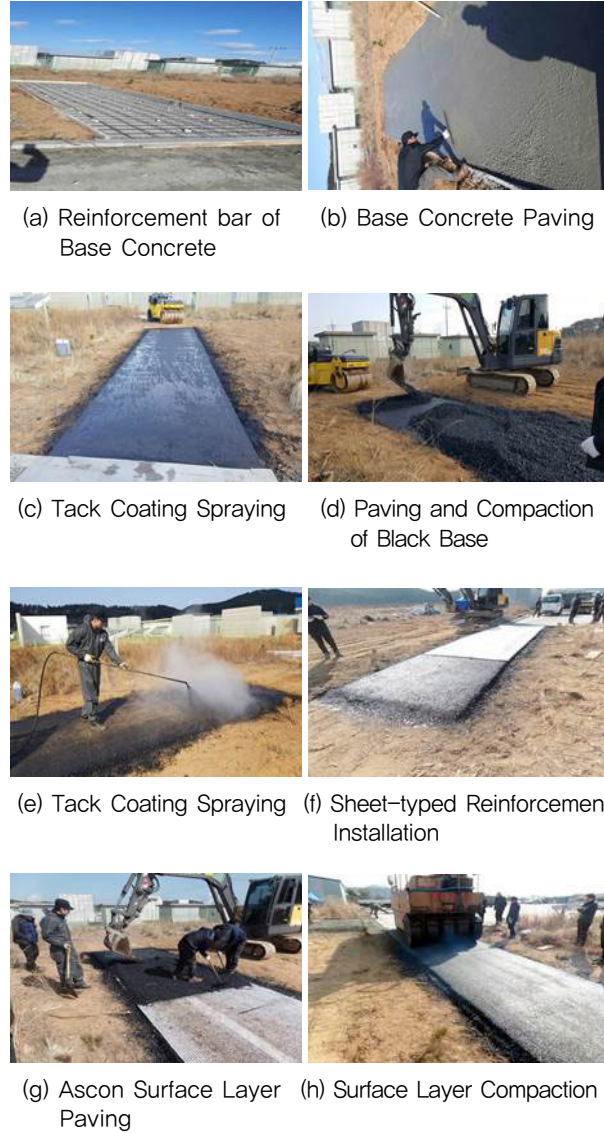
Fig. 14 Mock Up Construction Procedure
