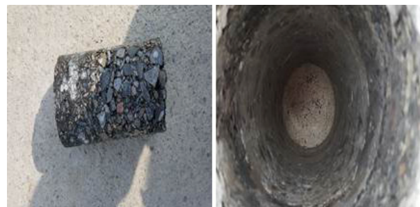
Fig. 16 Internal State of Mock Up Pavement Layer
