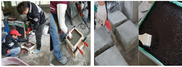
Production of RCC-Base & Curing 7days
