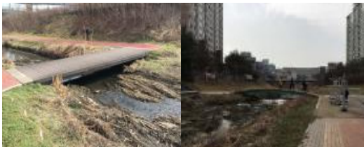
Fig. 8. Installation of a wooden bridge across the river
