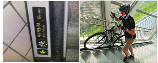
Fig. 9. Example of installation of bike ramp
