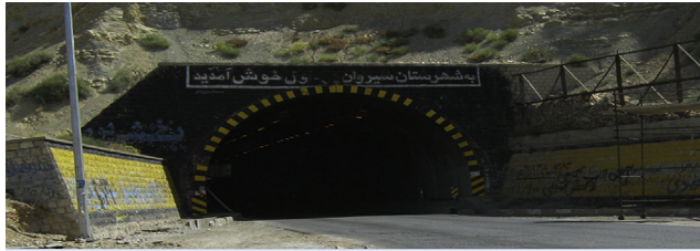
Fig. 1. Black hole phenomenon at the entrance to a road tunnel.
