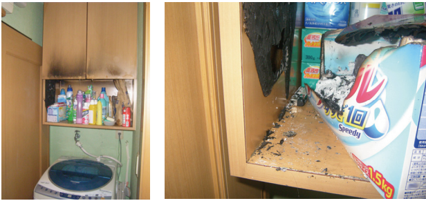
Figure 8. Fire case at shelf due to DGL.
