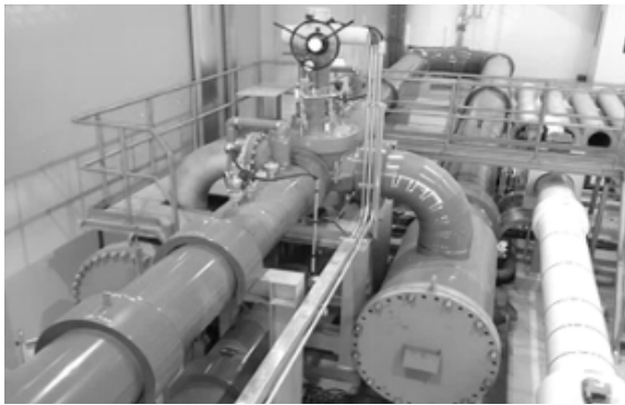
Fig. 7 Photograph of pipe prover
