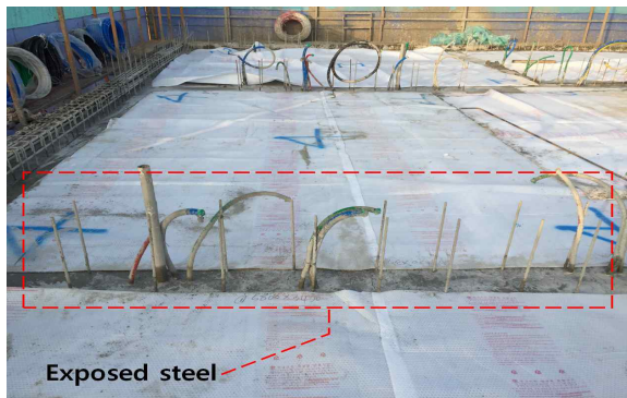
Figure 1. Picture of curing on the wall structure slab
