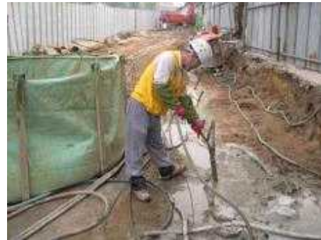
(b) Grouting method
