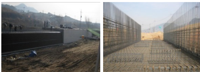
Fig. 4. Condition of excavation works for the New-Town utility tunnel(SMG, 2014)
