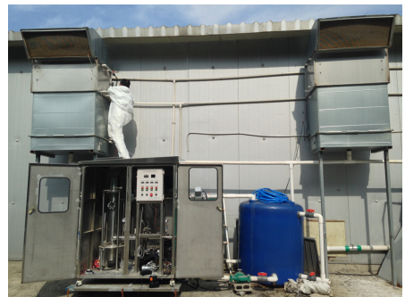
Figure 1. Schematic diagram of operation process(left) and on-site photo(right) of air cleaner applied to the pig house
