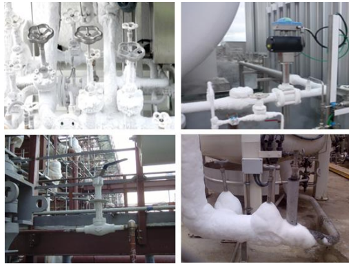
Fig. 1 Applications for cryogenic valves on LNG system
