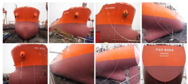
(c) Hull Condition after Redocking
