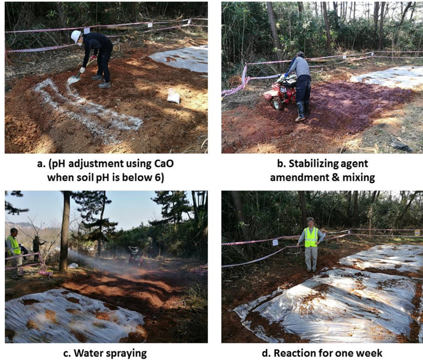
Fig. 5. Procedure for application of stabilizing agents in As-contaminated soil at the forest area near the former Janghang smelter site.
