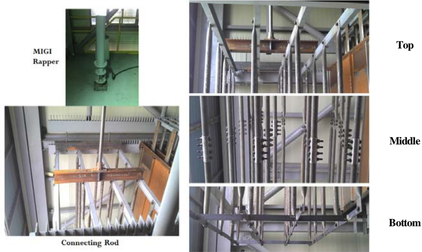
Fig. 3. Test setting at ESP test tower.
