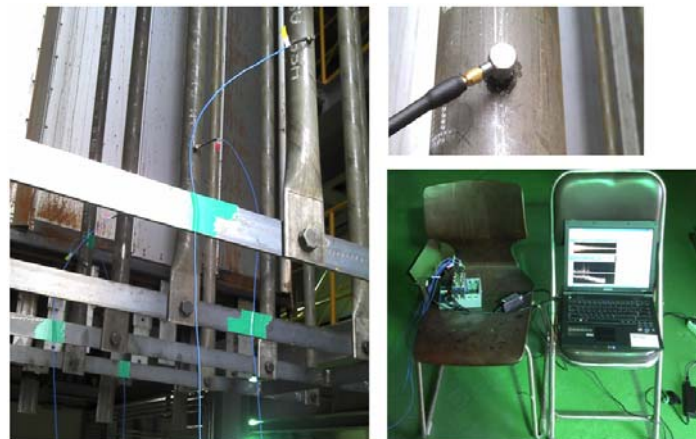
Fig. 2. Test setting for vibration data acquisition.
