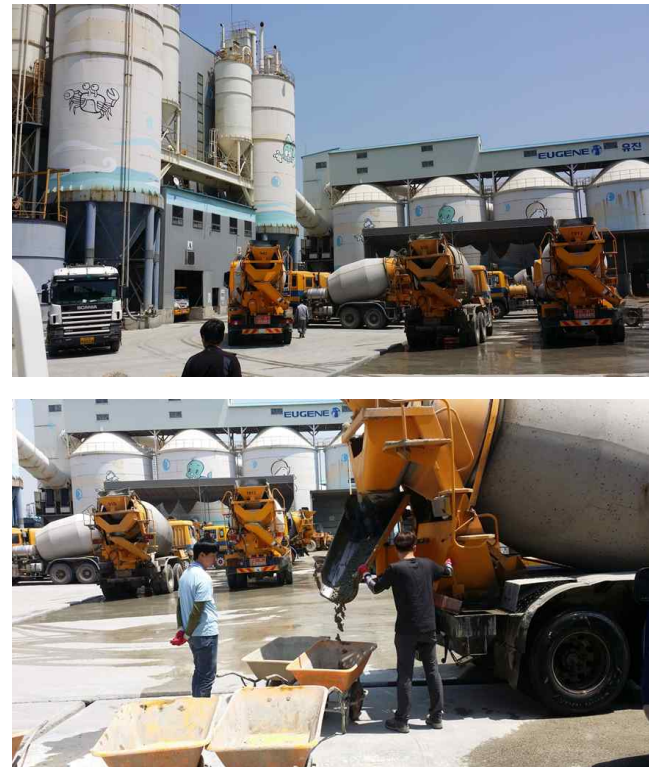
Figure 1. Ready-mixed concrete plant and manufacture
