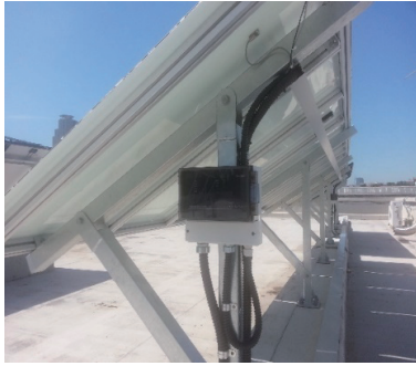
Fig. 3. The terminal box synthesized the measured value by each sensor.
