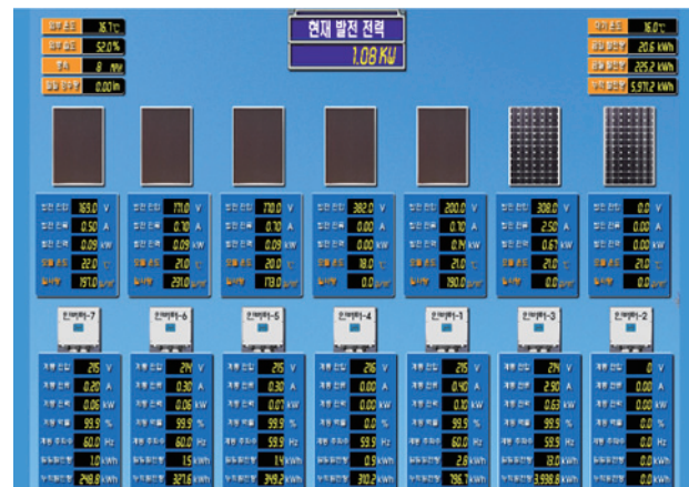
Fig. 2. Monitoring system installed on the roof of Konkuk University.
