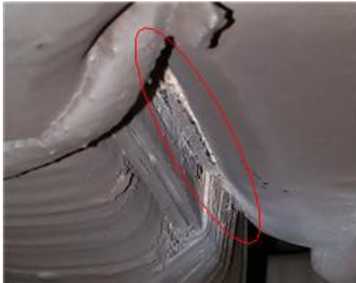
Fig. 3. Efflorescence of the terminal windings.
