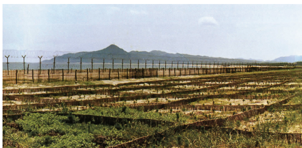
Figure 2. Hedges fixed during plantation in the east coast of Korea (sand dune fixation works with higher hedge and sand dune stabilizing works with lower hedge). (Hong, 2016)
