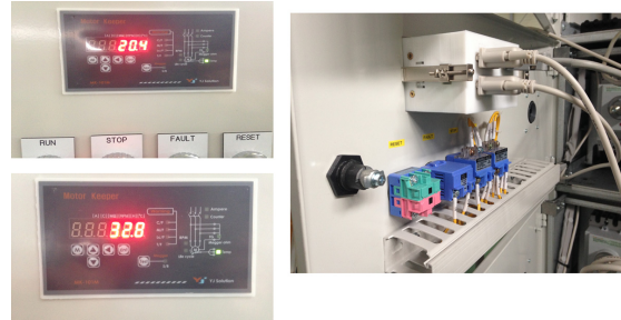
Fig. 12 Display busbar temperature on busbar monitor
