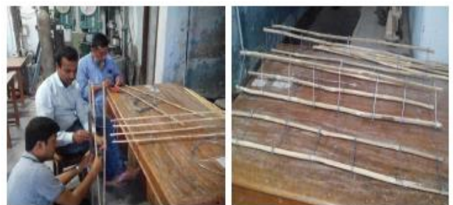
FIGURE VI Bamboo Reinforcement binding for Beam and Column Specimens
