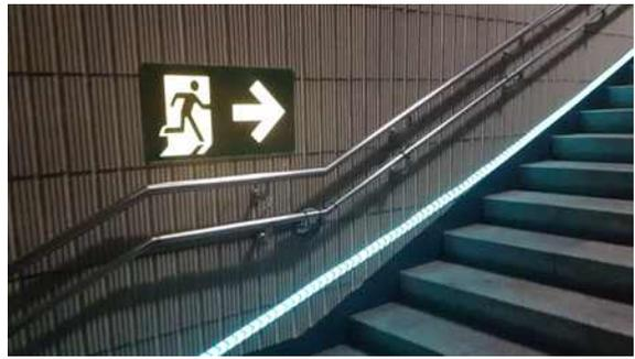
(b) Lower step type tape-shaped direction indicating EL display panel
