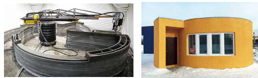
Fig. 5. 3D printing residential building (Apis-cor)
