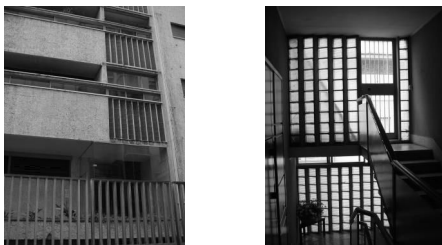
Figure 8. Exterior and interior view of stair tower
