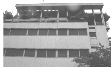
Figure 14. North facade's two balcony rails
