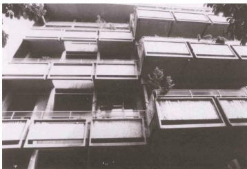
Figure 12. West facade: six window bays
