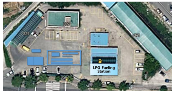
Fig. 3. Example of hydrogen multi energy filling station site research
